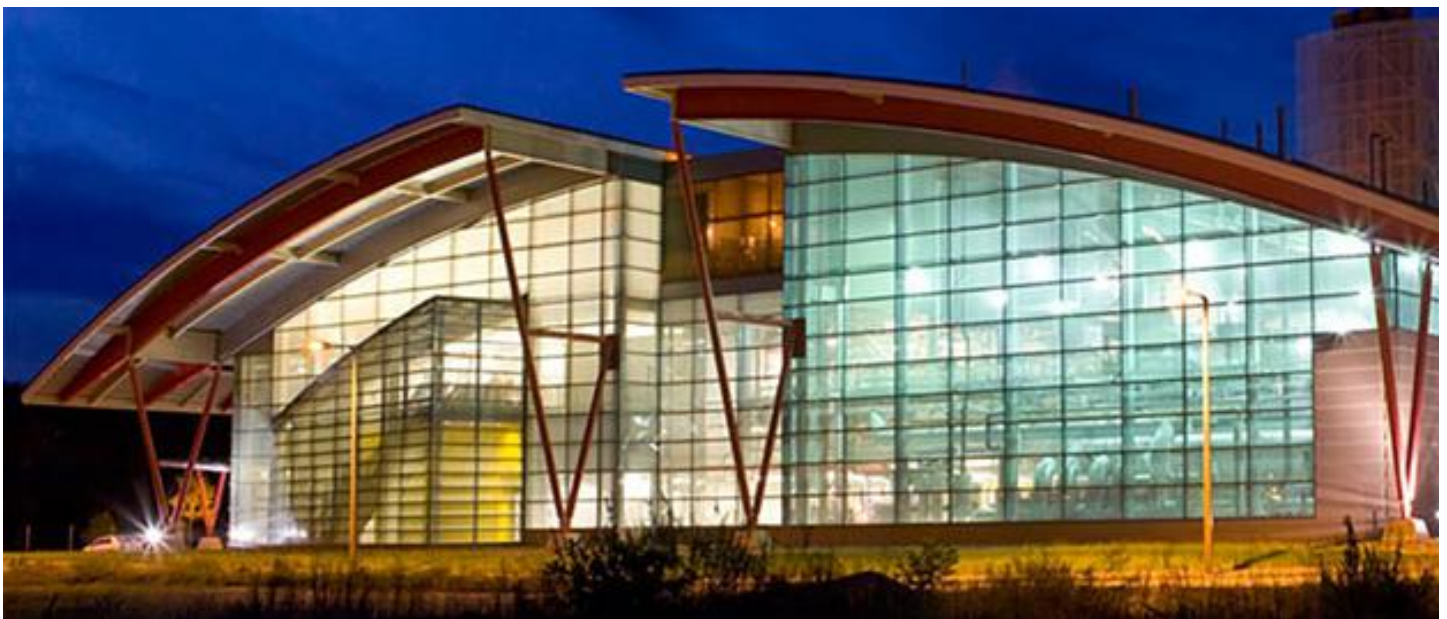
The University of Massachusetts Amherst Central Heating Plant, pictured above, provides 70% of the campus' electricity and 100% of its steam needs from natural gas. In the future, district heat systems such as this could operate using the dual-fuel approach that leverages electric boilers when renewable energy is abundant and low-carbon gas at other times. Photo credit: UMass Amherst
